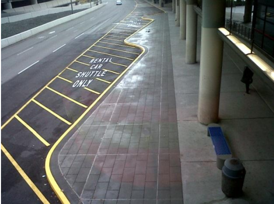
Sidewalk and Shuttle Stop Improvements
