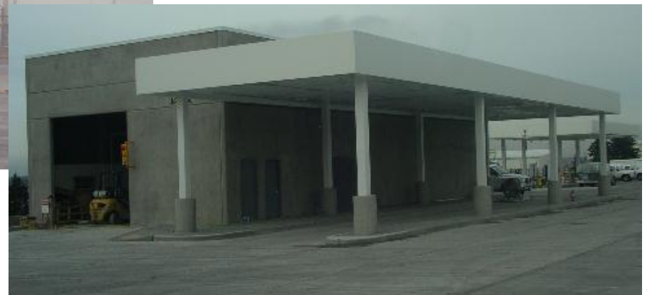
Bus Wash Facility
